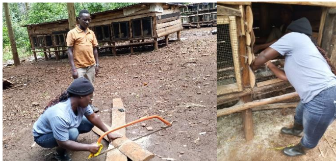
Figure 30. Renovating the Rabbit House
