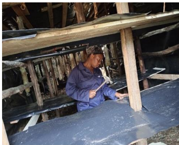
Figure 25.Renovating the mushroom house
