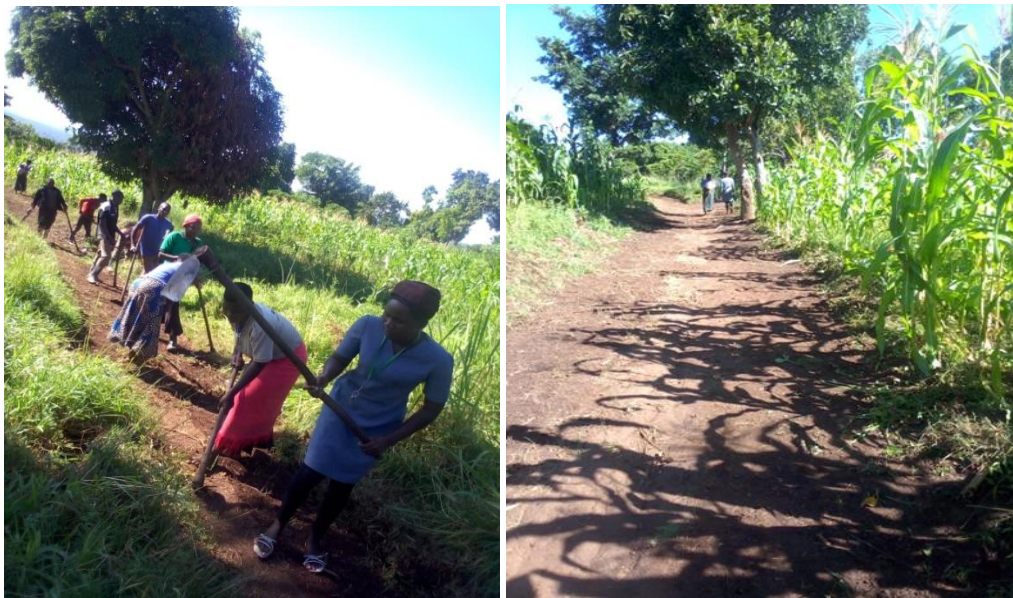
Figure 17: On the left Intern and Community members clearing the road and on the right is the cleared road
