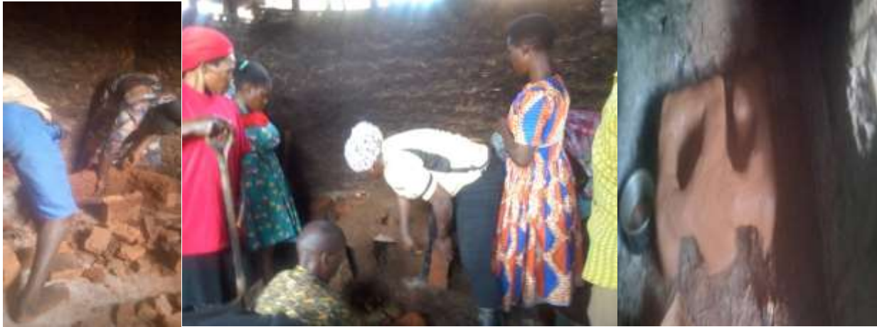
Photo 13: The Intern training Kisaara Members in constructing Lorena stoves
