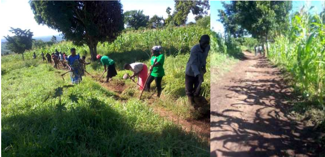
Photo 12: The Intern and community members clearing a 4km Kisaara-Kenga road
